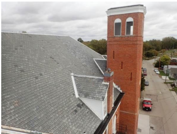
Roof – Overview of “C” – South Slope
