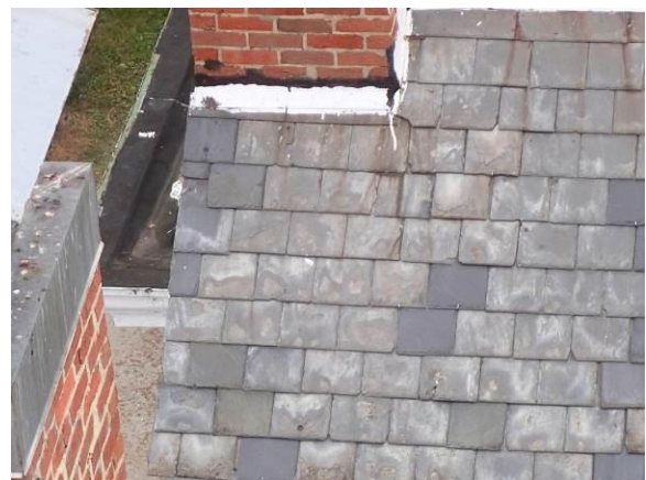
Roof – “Y” Slope – Missing at Rake Downslope of Chimney
