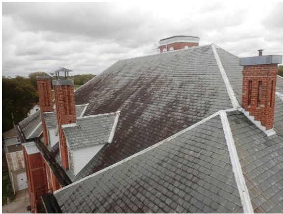
Roof – “O” Slope – Overview
