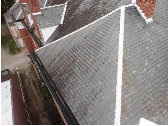
Roof – “M” Slope – Overview
