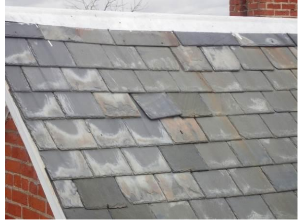
Roof – “K” Slope – Displaced Tile
