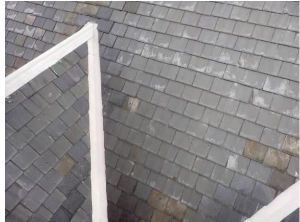
Roof – “D” Slope – Missing Tile near Valley
