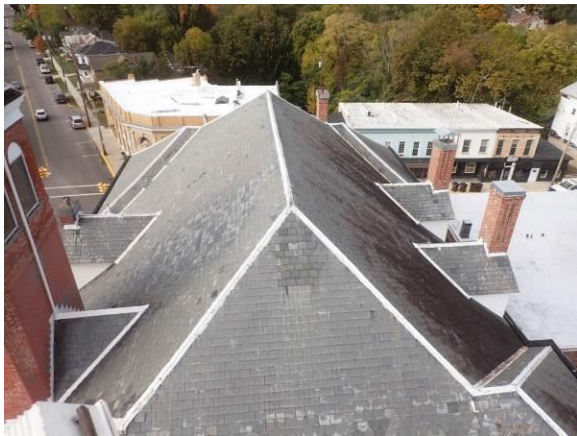
Roof – Overview – Looking West
