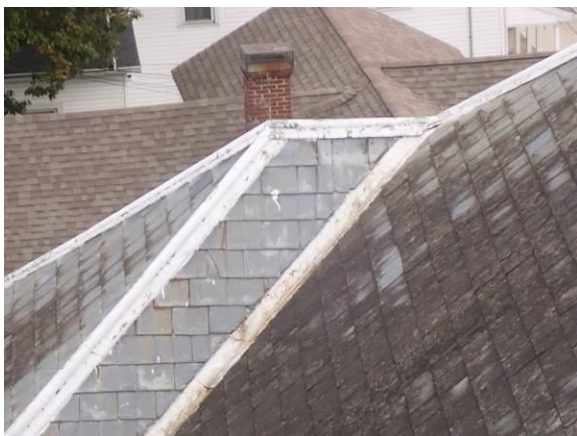
Roof – “L” Slope – Missing Tile near Ridge
