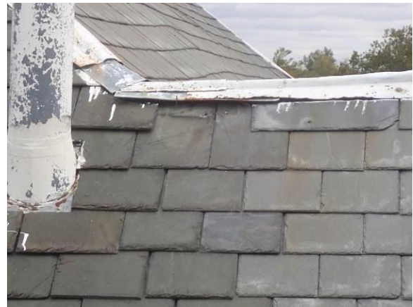
Roof – “J” Slope – Missing Tile near Ridge
