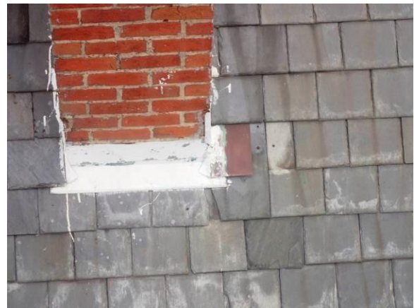
Roof – “J” Slope – Missing Tile near Chimney Penetration
