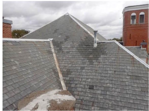
Roof – Replacement Tiles on West Slope
